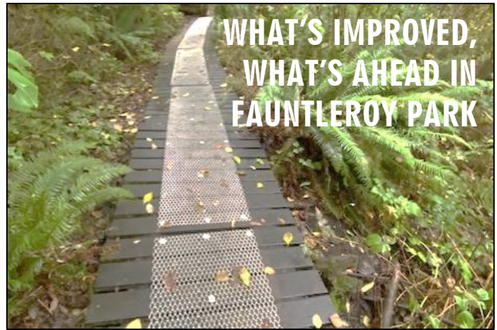
Seattle Parks improved visitor safety by upgrading the wire mesh on 150 feet of boardwalk in Fauntleroy Park. Photo courtesy Tom Trulin
