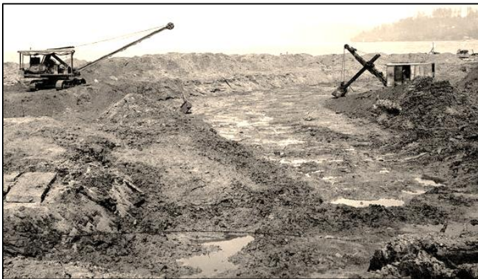
Steam power did the heavy work to scoop out the pool. Seattle Municipal Archives # 28725
