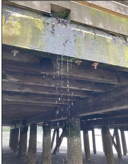
**Upgrading the ferry terminal will include installing a state-of-the-art collection system for pollutants now running off the dock into Fauntleroy Cove.** Photo by Chuck Sawyer
