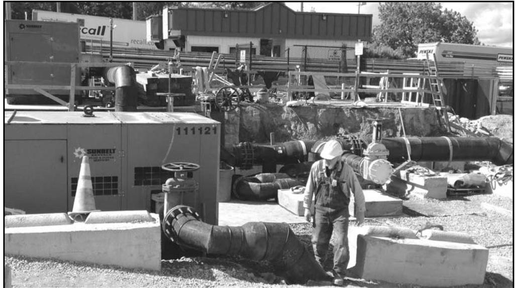
**Prospect Construction has finished installation of bypass piping and two standby diesel pumps to serve during while underground work proceeds.** *Photo courtesy King County Wastewater*
