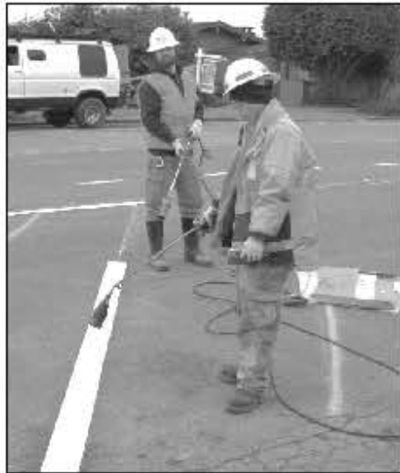
A crew redid cross-hatching in January 2014. Photo courtesy PhilSweetland
