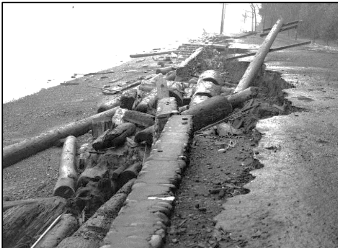
Storm damage in 1951 seriously damaged the south seawall and promenade. Courtesy Seattle Municipal Archives, #42581
