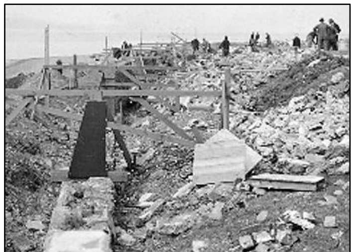
(Above) Strong backs, augmented by horsepower, had the seawall well under way in 1934. (Below) Two years later, construction was nearing Point Williams. Courtesy Seattle Municipal Archives, #29742, #29700
