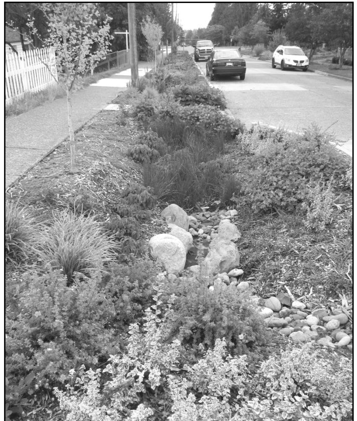
This half block-long roadside rain garden in Sunrise Heights/Westwood is off to a good start. Photo courtesy Seattle Public Utilities
