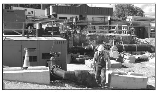
Prospect Construction has finished installation of bypass piping and two standby diesel pumps to serve during while underground work proceeds. Photo courtesy King County Wastewater
