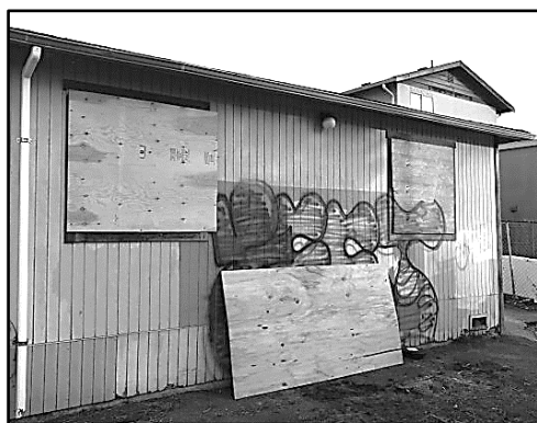
Fire took this derelict West Seattle house to the ground in 2017 after squatters had caused two prior blazes. Photo courtesy West Seattle Blog
